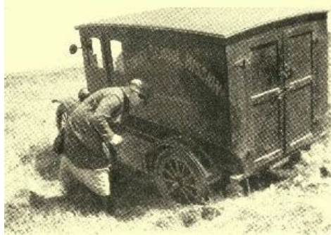
DIGGING OUT THE WHEEL
