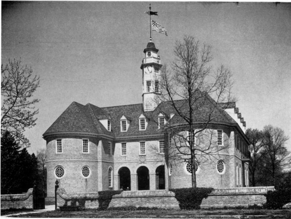
The Old Capitol at Williamsburg, showing the north elevation which is a duplicate of the historic Virginia Capitol originally completed in 1705. Courtesy of Colonial Williamsburg, Inc.
