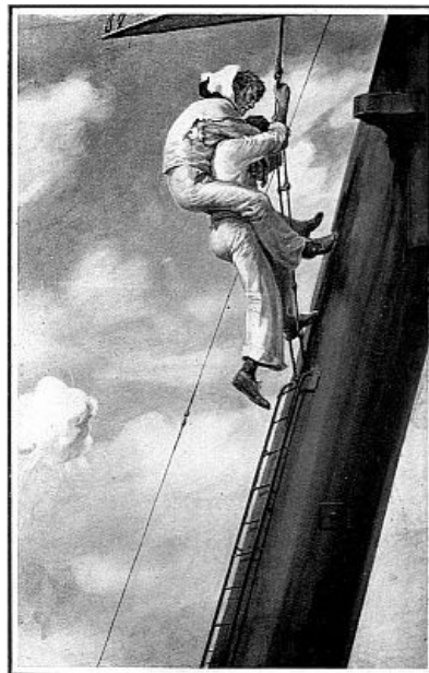
THE TRIPOD MAST.
