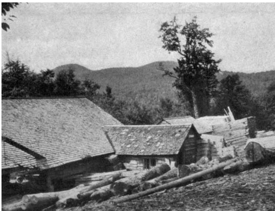
Owl's Head over the roof of the saw mill
