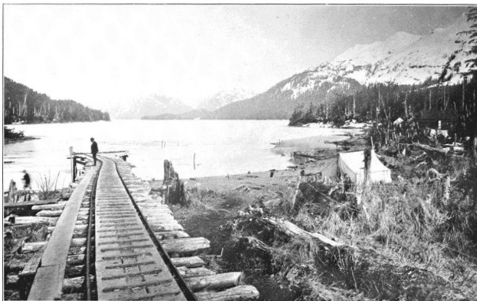
Copyright by E. A. Hegg, Juneau Railroad Construction, Eyak Lake
