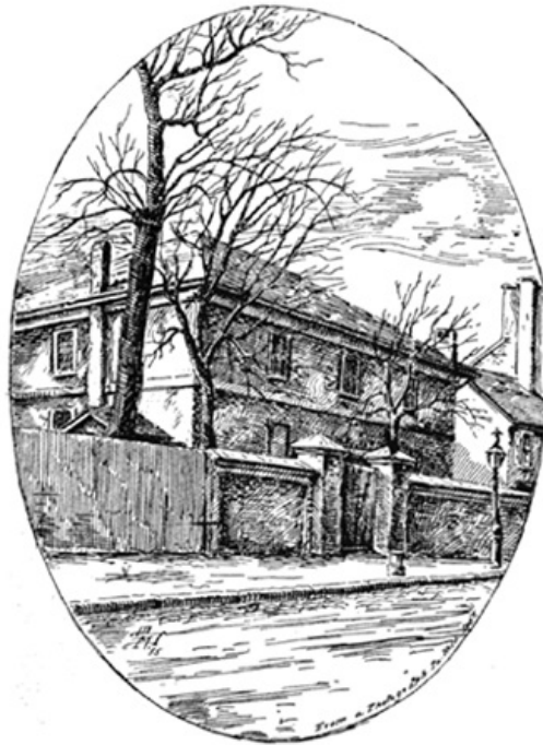
Pine Street Meeting-House. Built 1751.
