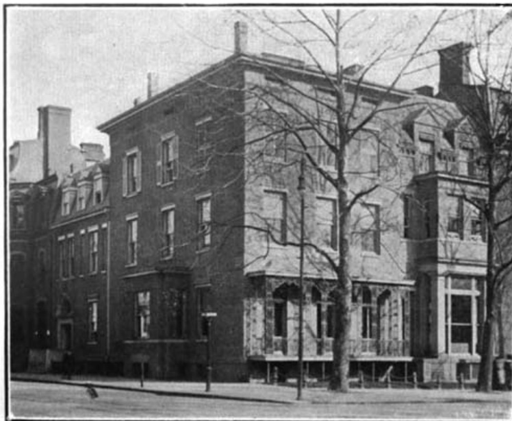
Madison House, Washington, D. C., West View. Photographed by Samuel M. Brosius.
