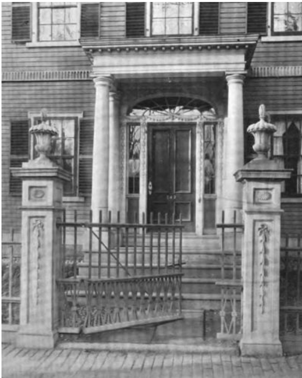
PLATE> II.—Doorway, Oliver House, Salem, Mass. Built in 1802.
