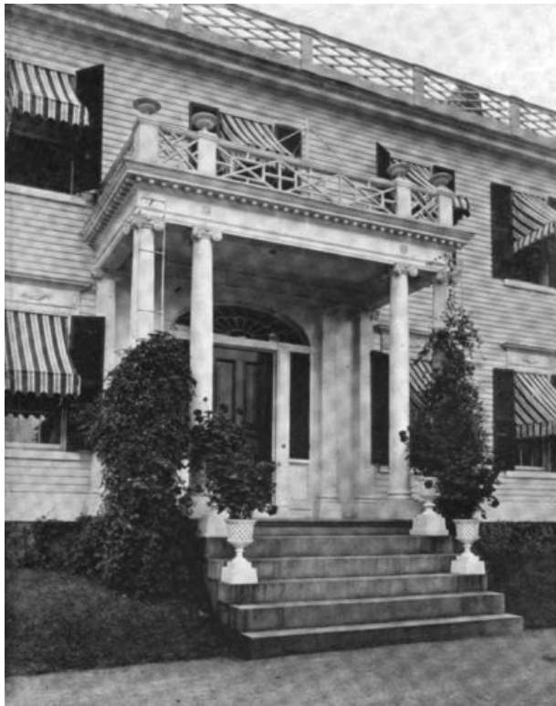
PLATE XXII.—Doorway, Rogers House.
