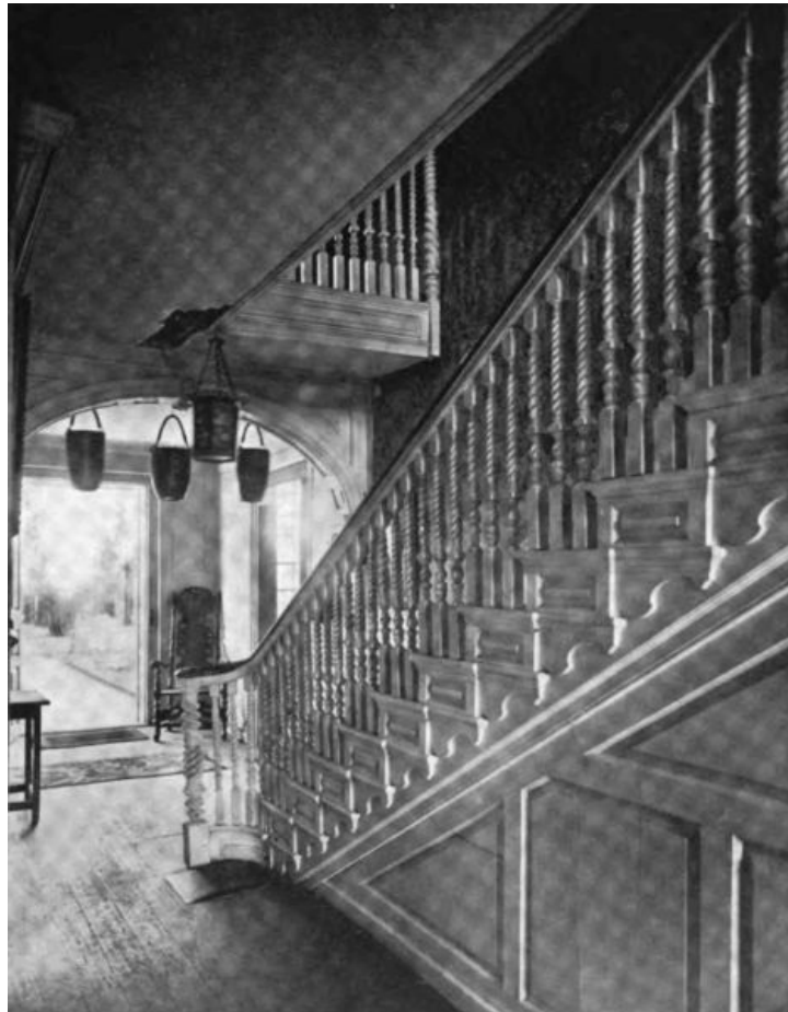
PLATE LXXX.—Hallway from the Rear, Royall House.
