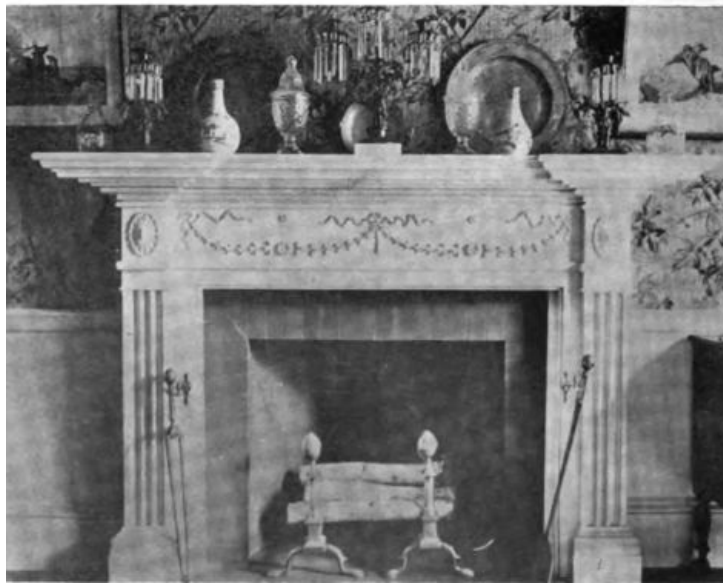
PLATE LXXVII.—Soapstone Fire Frame, Kittredge House Fireplace, Kittredge House.
