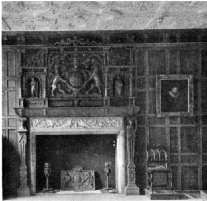
FIREPLACE AND OAK PANELLING FROM THE "OLD PALACE" AT BROMLEY-BY-BOW. BUILT IN 1606.
