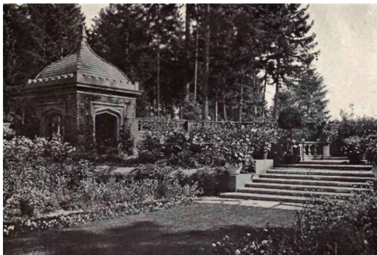
PLATE 176 "Thornewood," Tacoma, Wash. Chester Thorne, Esq.
