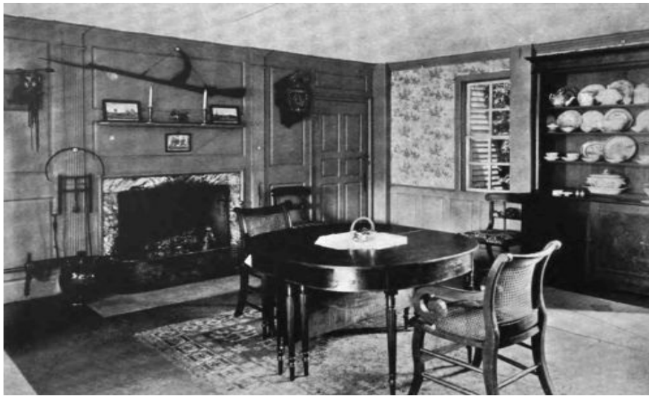
Plate XVII.—Old Fireplace in Wentworth House, Portsmouth, N. H.
