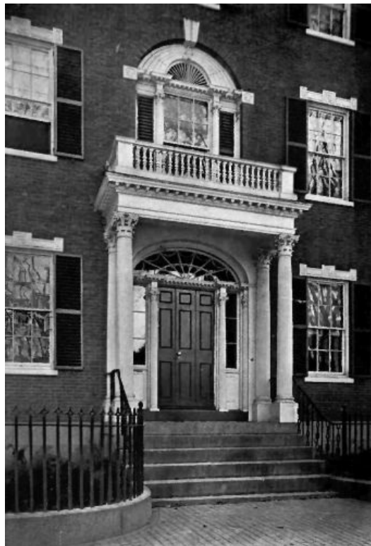
Plate I.—Dodge-Shreves Doorway. Built in 1816.
