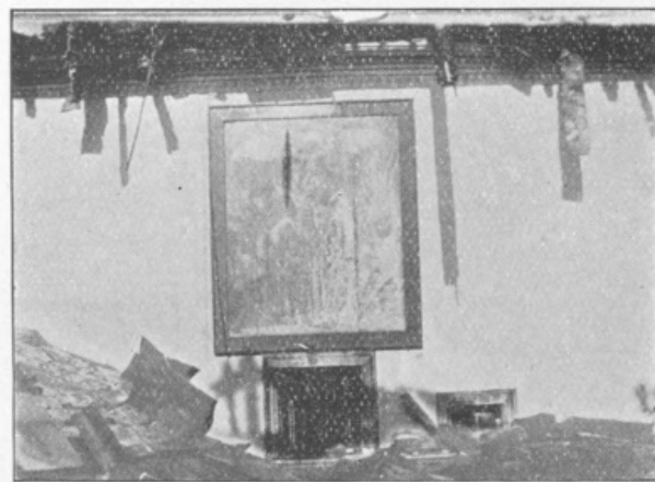
COURT ROOM AFTER THE FIRE.
