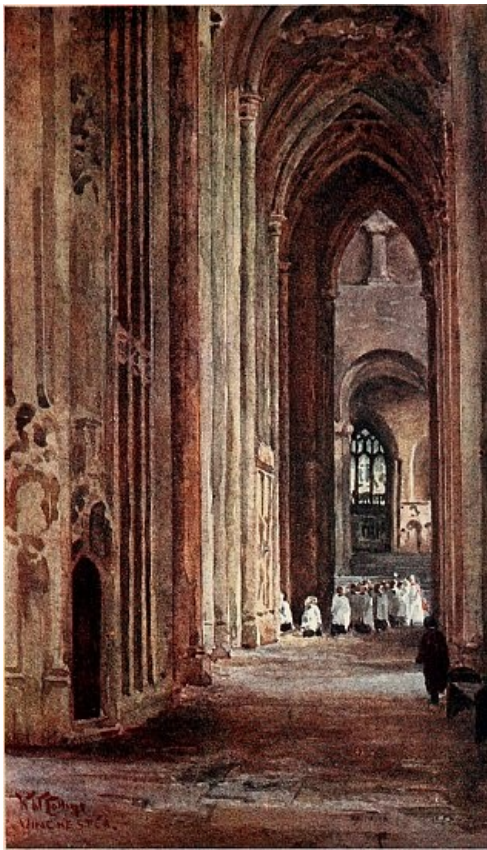
WINCHESTER THE NORTH AISLE
