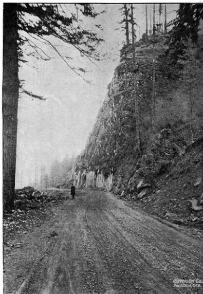
ON THE COLUMBIA RIVER HIGHWAY IN HOOD RIVER COUNTY TWO MILES EAST OF CASCADE LOCKS. GRADED AND GRAVELED IN 1917 AND 1918
