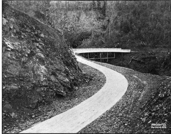
ON THE PACIFIC HIGHWAY SOUTH OF WOLF CREEK IN JOSEPHINE COUNTY. CONSTRUCTED IN 1917 AND 1918
