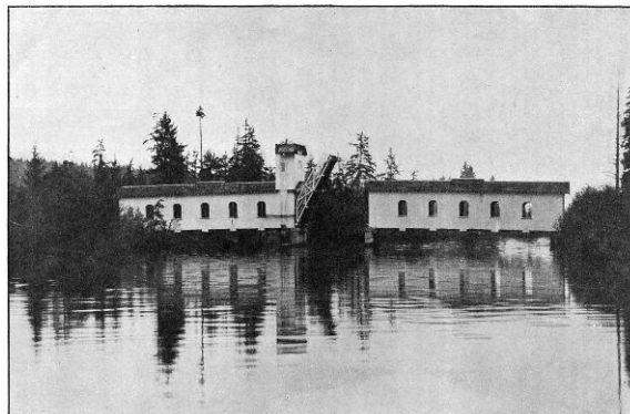
COVERED WOOD DRAWBRIDGE ON THE COLUMBIA RIVER HIGHWAY IN CLATSOP COUNTY, OVER THE JOHN DAY RIVER EAST OF ASTORIA. BUILT IN 1918. LIFT SPAN—40 FEET
