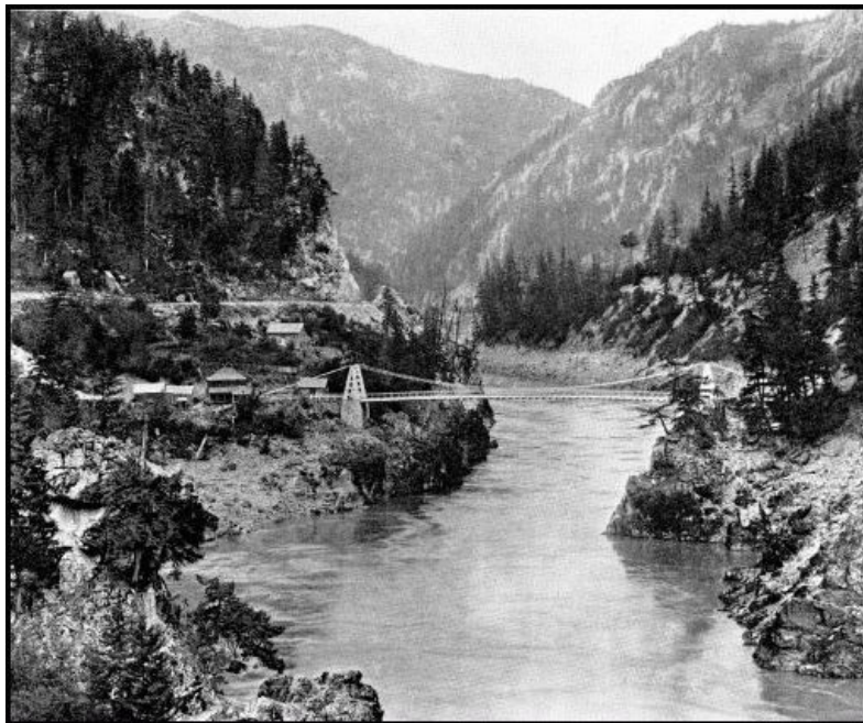
CARIBOO ROAD BRIDGE, FRASER CANYON
