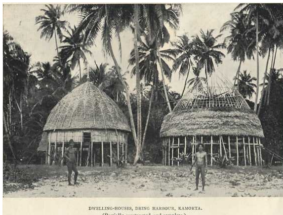
DWELLING-HOUSES, DRING HARBOUR, KAMORTA. (Partially constructed, and complete.)
