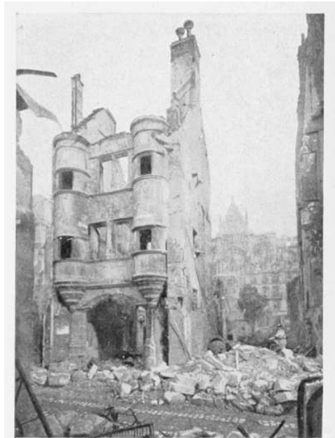
DOOR OF THE CHAPTER-HOUSE COURTYARD
