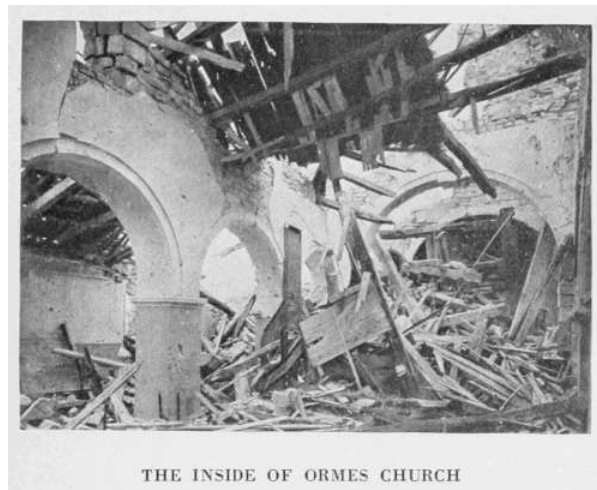
THE INSIDE OF ORMES CHURCH
