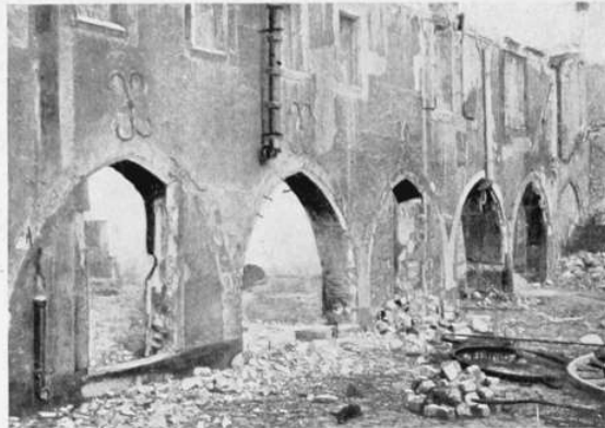
INTERIOR FAÇADE OF THE CLOISTER OF THE FRANCISCAN FRIARS In the courtyard of No. 9, Rue des Trois-Raisinets.
