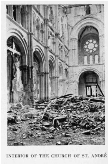
INTERIOR OF THE CHURCH OF ST. ANDRÉ
