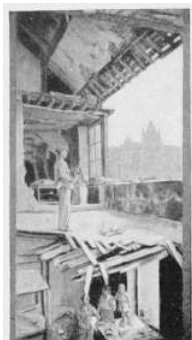
THE FIRST AND SECOND STORIES OF A HOUSE IN THE RUE D'ANJOU, AFTER THE BURSTING OF AN 8-IN. SHELL
