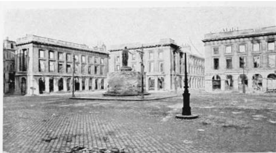
THE PLACE ROYALE IN 1918 The plinth of the statue was protected by masonry-work.
