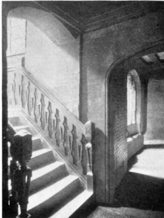
STAIRCASE LEADING TO CLOISTER GALLERY.
