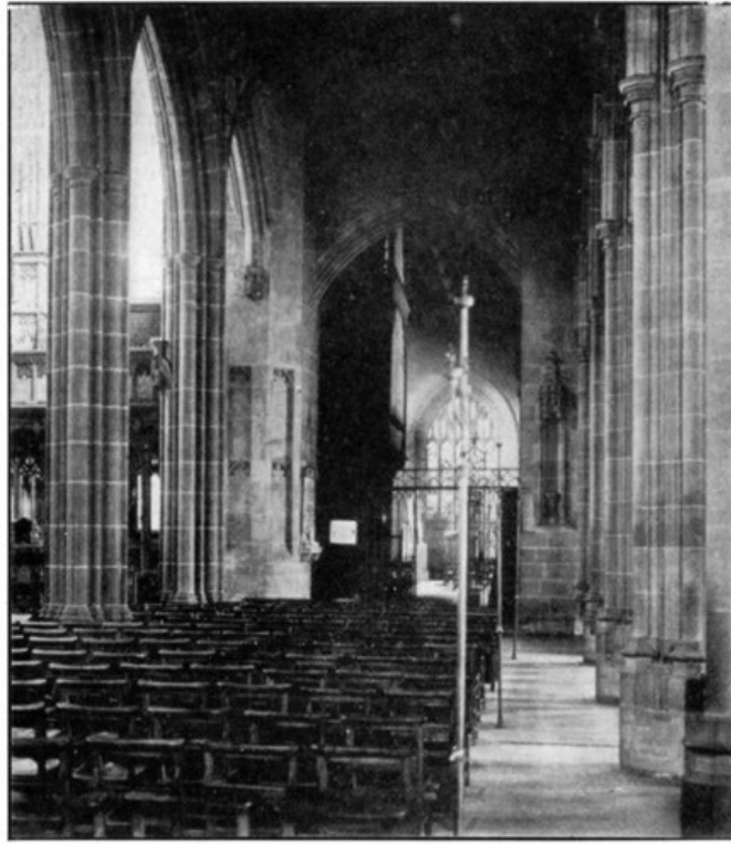
THE INNER SOUTH AISLE OF THE NAVE.
