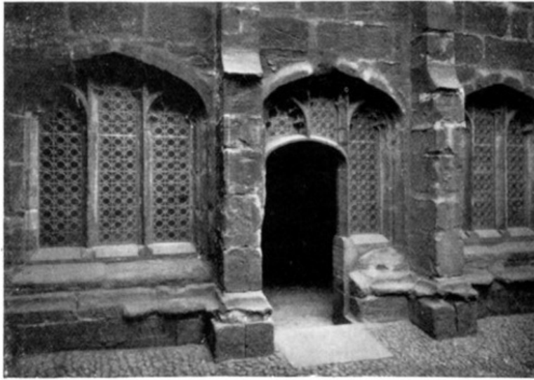
WEST SIDE OF THE CLOISTER.
