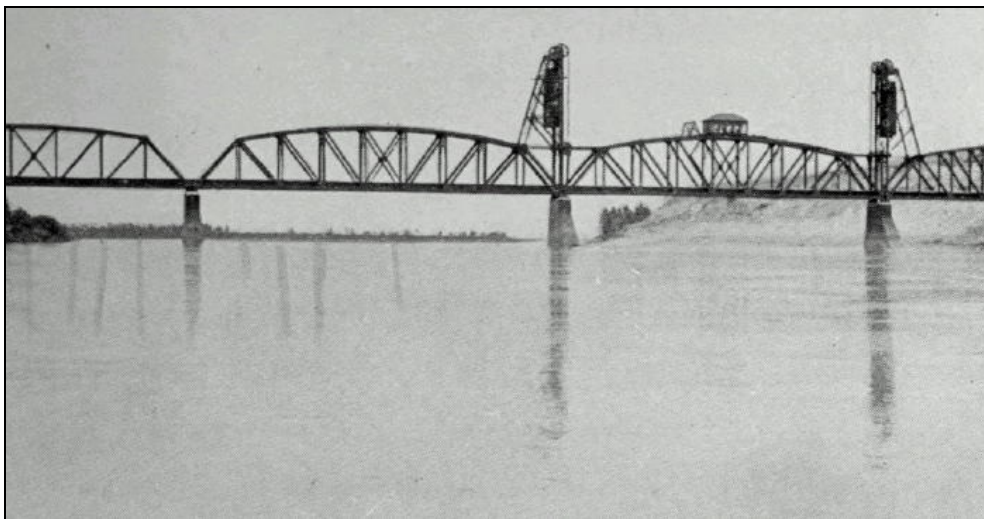
THE LAST BRIDGE ABOVE THE MISSOURI
