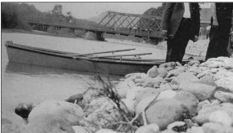
WE LAUNCHED THE BOAT BELOW THE LIVINGSTON BRIDGE
