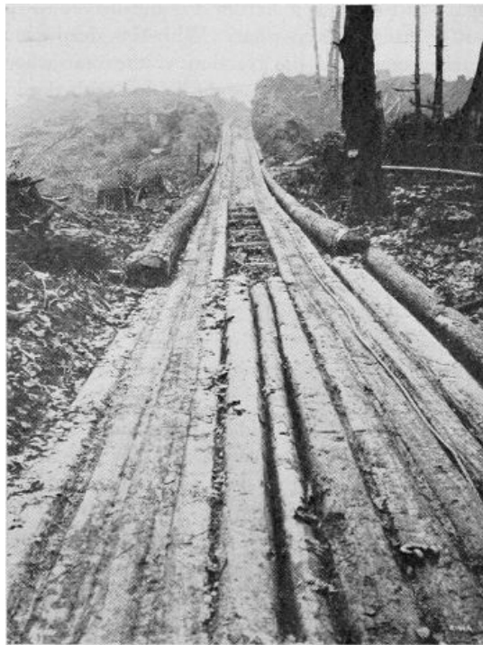
The most common type of motor truck logging road— a fore-and-aft pole road.
