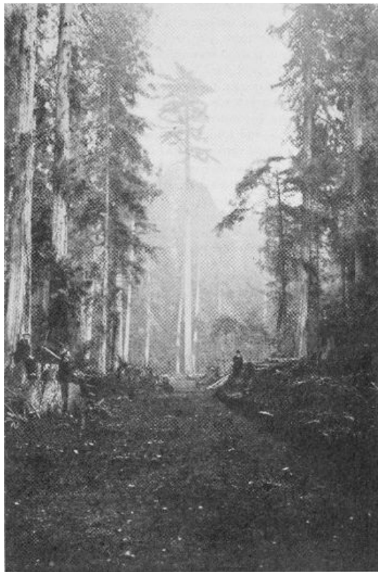
Sub-grade for motor truck logging road.
