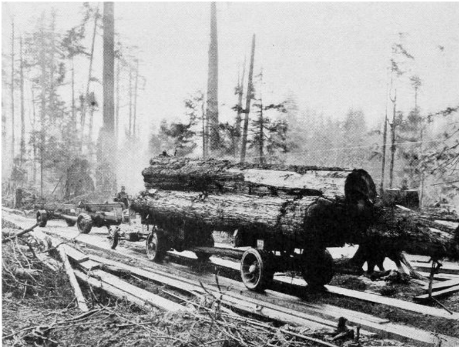
Turn out on fore-and-aft plank road.
