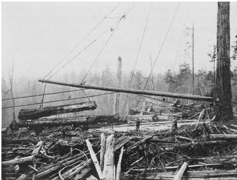
Loading a motor truck and trailer through the use of a boom.
