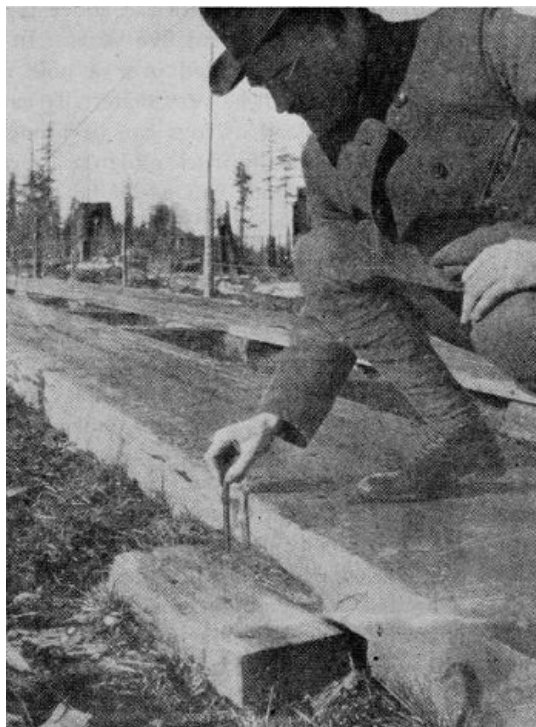
Detailed view of fore-and-aft plank road, showing method of wedging.
