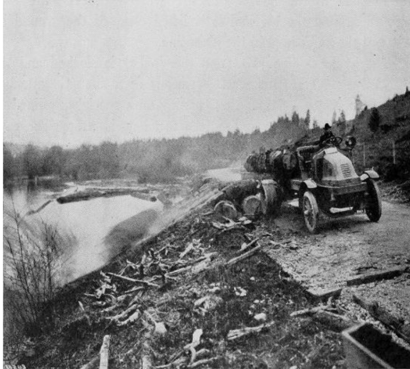
Unloading truck and trailer through the use of an incline, showing brow-skids and roll-way.
