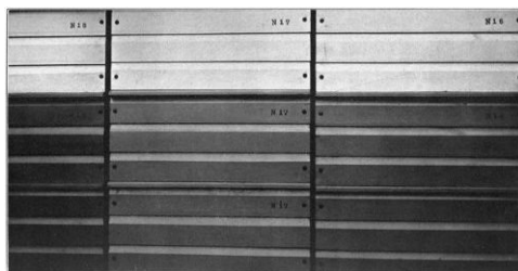
Section of Fence Showing New Panels Recently Placed
