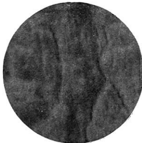
9. Formula No. 24, Panel 36, on 1907 Fence. Good Condition. Surface Checking Only
