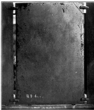
Corroded and Pitted Surface of Plate Painted with Stimulative Paint
