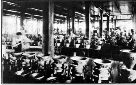
Batteries of Color Grinding Mills
