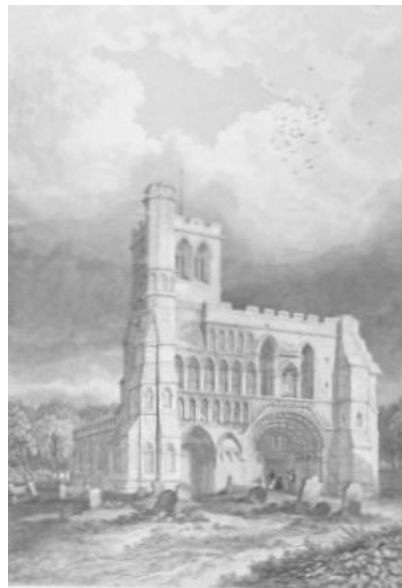
DUNSTABLE PRIORY CHURCH, (WEST FRONT.) BEDFORDSHIRE.
