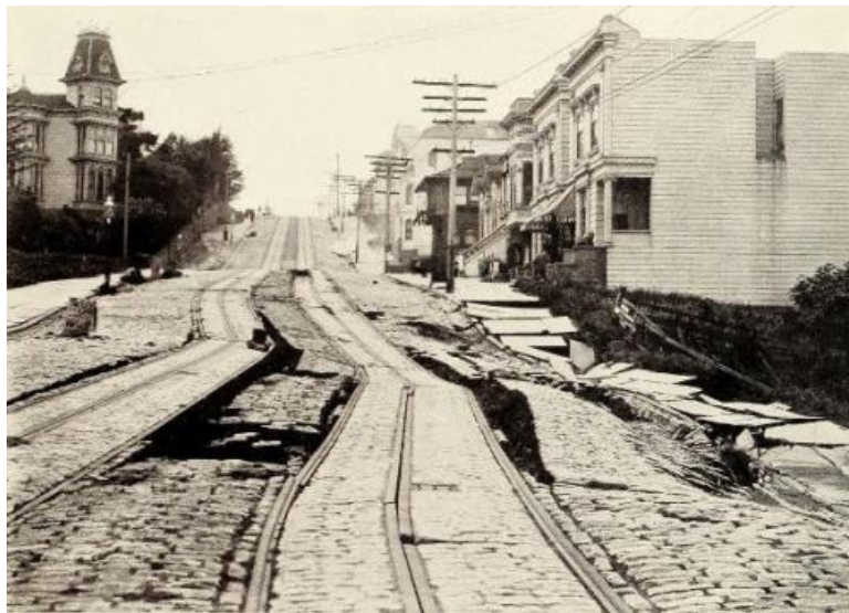
Section of the Union Street Cable Line, Between Steiner and Pierce Streets, Distorted by the Earthquake.
