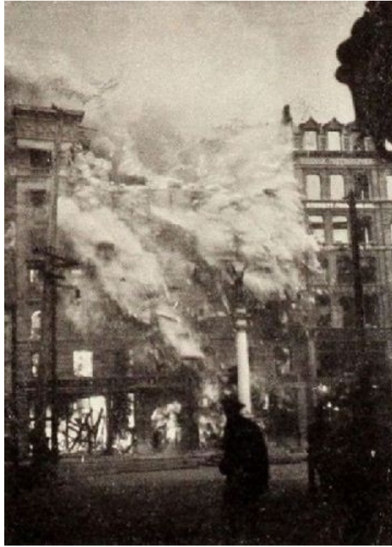
Destruction of the Emma Spreckels Building, on the First Floor of Which Was "Zinkands."
