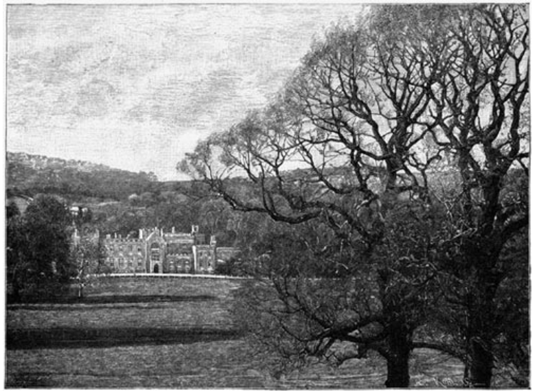
West Dean. Example of country seat in which terracing is needless, and in which turf may and indeed must often come to at least one side of the house
