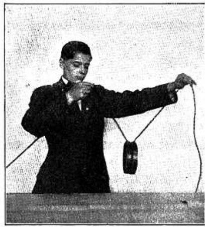
FIG. 24—TWO COILS WITH CURRENTS FLOWING IN SAME DIRECTION ATTRACT EACH OTHER
