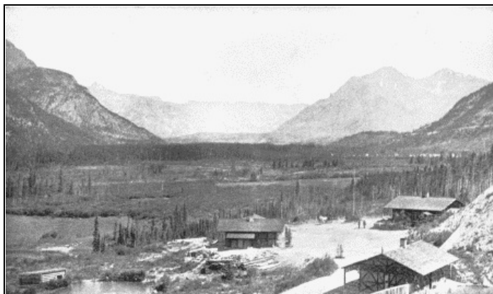
MINING CAMP IN NEVADA.
