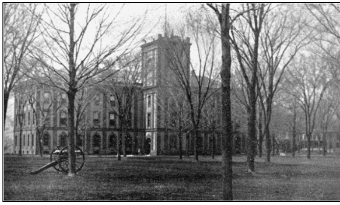
THE SPRINGFIELD ARMORY.
