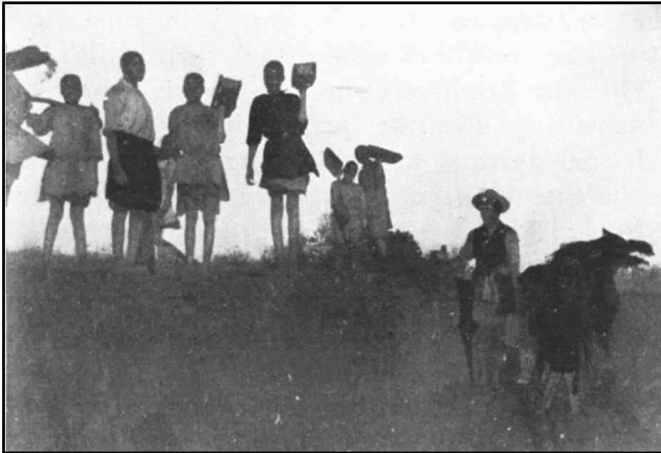
Making Brick at Macha.
