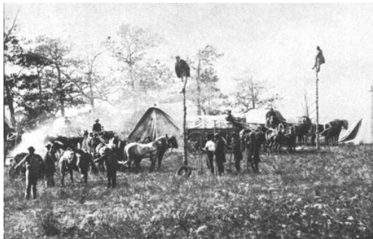
The Union military telegraph corps strung more than 15,000 miles of wire during the war. In one year, the Northern armies kept the wires alive with nearly 1.8 million messages. Galvanic batteries transported by wagon furnished the electricity.
