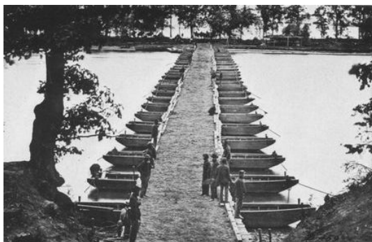
General Lee had hoped that Virginia's numerous streams and rivers would delay Grant's advance, but Federal engineers with portable pontoon bridges kept the army at Lee's heels.
