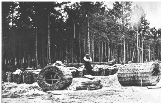
Gabions, open-end baskets filled with earth, proved as effective as masonry in defensive works. Thousands of these baskets were patiently made by hand for use in field and seacoast fortifications.
