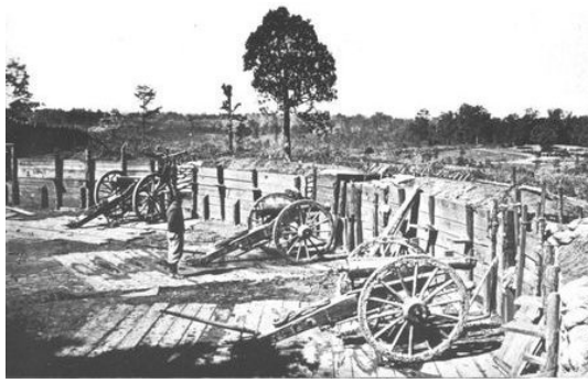
Confederate sappers constructed a number of artillery emplacements covering the avenues of approach to Atlanta. The guns in this fortification overlook famous Peachtree Street.
