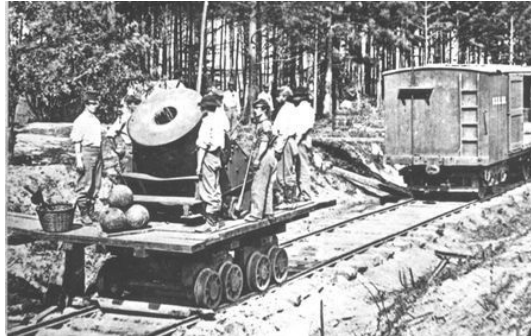
Moved by special rail to the Petersburg front, the 13-inch mortar "Dictator" hurled 200-pound exploding shells at the Confederate earthworks over two miles away.
