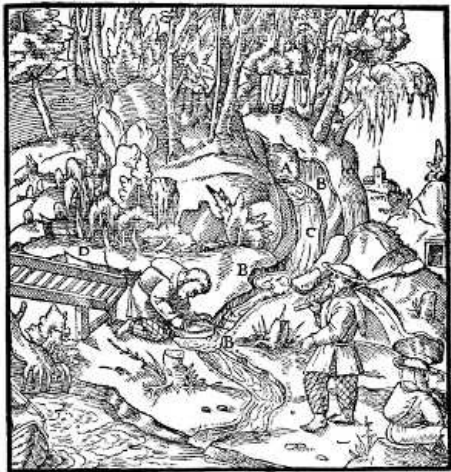
A—GULLY. B—DITCH. C—TORRENT. D—SLUICE BOX EMPLOYED BY THE LUSITANIANS. [Pg 347]
