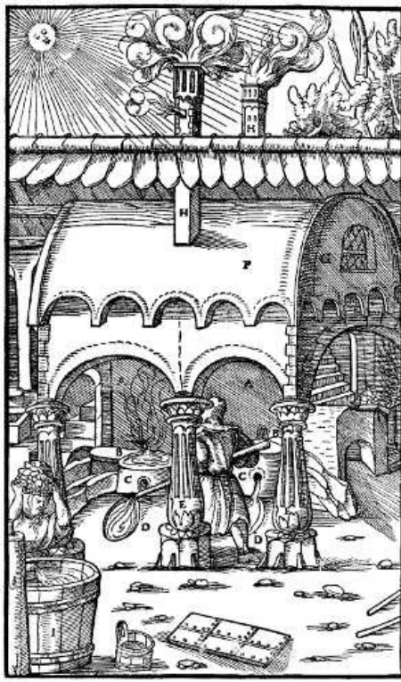
A—FURNACES. B—FOREHEARHS. C—THEIR TAP-HOLES. D—DIPPING-POTS. E—PILLARS. F—DUST-CHAMBER. G—WINDOW. H—CHIMNEYS. I—TUB IN WHICH THE COALS ARE WASHED. [Pg 417]
