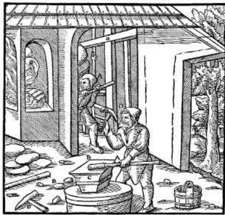
A—POINTED BAR. B—THIN COPPER LAYER. C—ANVIL. D—HAMMER. [Pg 534]
