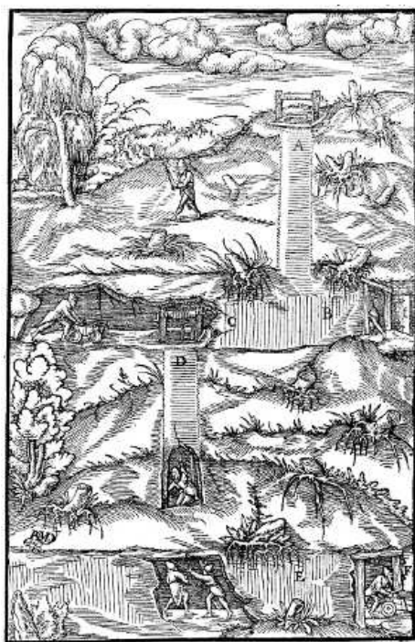
A—SHAFT. B, C—DRIFT. D—ANOTHER SHAFT. E—TUNNEL. F—MOUTH OF TUNNEL. [Pg 105]
