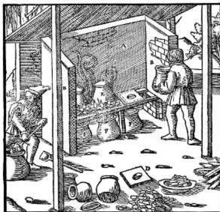
A—LONG WALL. B—HIGH WALLS. C—LOW WALLS. D—PLATES. E—UPPER POTS. F—LOWER POTS. [Pg 581]
