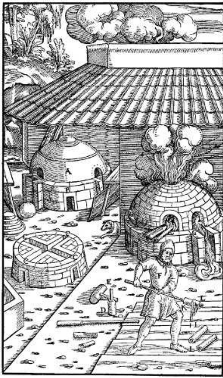
A—CHAMBER OF THE FURNACE. B—ITS BED. C—PASSAGES. D—RAMMER. E—MALLET. F—ARTIFICER MAKING TUBES FROM LITHARGE ACCORDING TO THE ROMAN METHOD. G—CHANNEL. H—LITHARGE. I—LOWER CRUCIBLE OR HEARTH. K—STICK. L—TUBES. [Pg 481]
