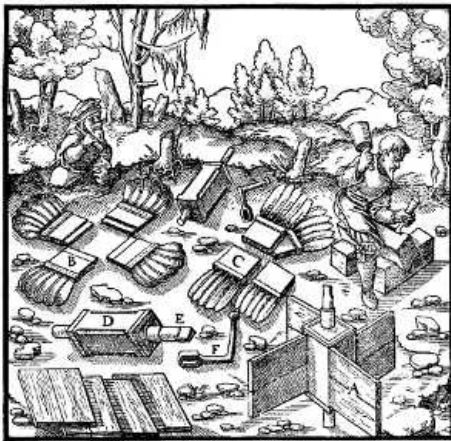
A—FIRST KIND OF FAN. B—SECOND KIND OF FAN. C—THIRD KIND OF FAN. D— QUADRANGULAR PART OF AXLE. E—ROUND PART OF SAME. F—CRANK. [Pg 207]
