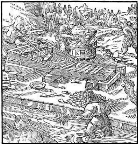
A—HEAD OF FRAME. B—SMALL LAUNDER THROUGH WHICH WATER FLOWS INTO HEAD OF FRAME. C—PIECES OF TURF. D—TROUGH PLACED UNDER FRAME. E—TUB IN WHICH PIECES OF TURF ARE WASHED. [Pg 333]
