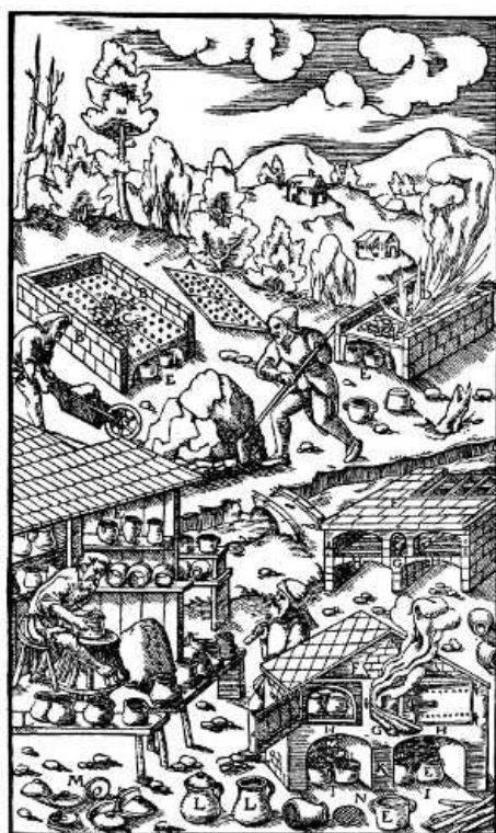
A—IRON PLATES FULL OF HOLES. B—WALLS. C—PLATE ON WHICH ORE IS PLACED. D—BURNING CHARCOAL PLACED ON THE ORE. E—POTS. F—FURNACE. G—MIDDLE PART OF UPPER CHAMBER. H—THE
