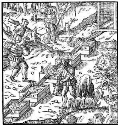
A—MOUTH OF THE TUNNEL. B—TROUGH. C—TANKS. D—LITTLE TROUGH. [Pg 585]
