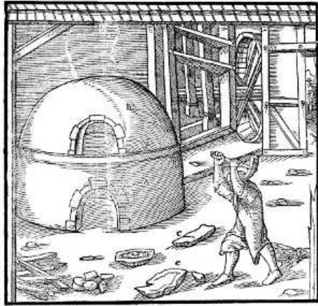
A—LOWER CHAMBER OF THE FIRST FURNACE. B—UPPER CHAMBER. C—VITREOUS MASS. [Pg 587]
