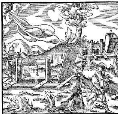
A—PROJECTING MOUTH OF CONDUIT. B— PLANKS FIXED TO THE MOUTH OF THE CONDUIT WHICH DOES NOT PROJECT. [Pg 202]
