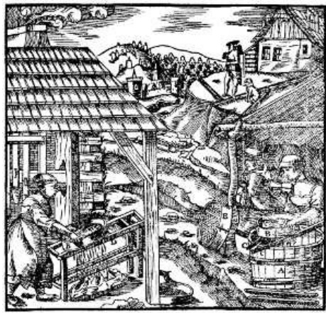
A—TUB. B—SIEVE. C—RODS. D—BENCH-FRAME. [Pg 374]
