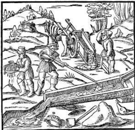
A—TROUGH. B—LAUNDER. C—HOE. D—SIEVE. [Pg 348]
