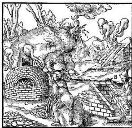
A—BURNING PYRE WHICH IS COMPOSED OF LEAD ORE WITH WOOD PLACED ABOVE IT. B—WORKMAN THROWING ORE INTO ANOTHER AREA. C—OVEN-SHAPED FURNACE. D—OPENINGS THROUGH WHICH THE SMOKE ESCAPES. [Pg 276]
