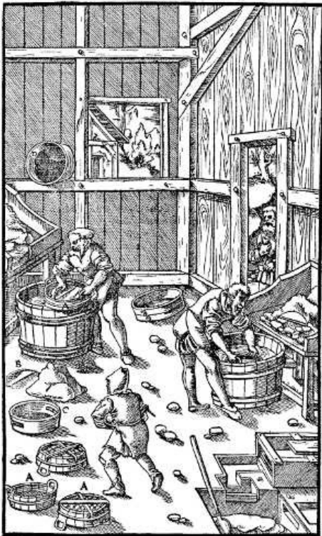
A—FINE SIEVES. B—LIMP. C—FINER SIEVE. D—FINEST SIEVE. [Pg 311]
