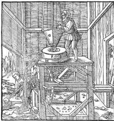
A—AXLE. B—WATER-WHEEL. C—TOOTHED DRUM. D—DRUM MADE OF RUNDLES. E—IRON AXLE. F—MILLSTONE. G—HOPPER. H—ROUND WOODEN PLATE. I—TROUGH. [Pg 294]
