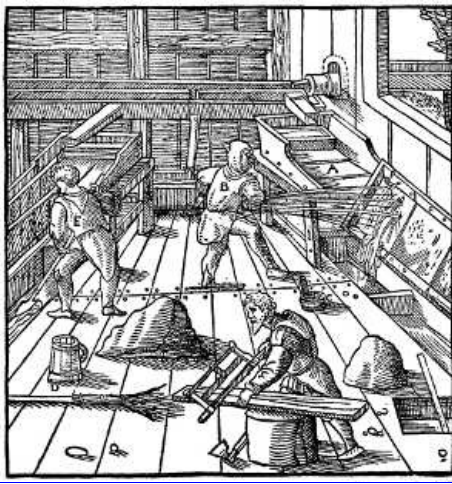
A—CANVAS STRAKE. B—MAN DASHING WATER ON THE CANVAS. C—BUCKET. D—BUCKET OF ANOTHER KIND. E—MAN REMOVING CONCENTRATES OR TIN-STONE FROM THE TROUGH. [Pg 309]
