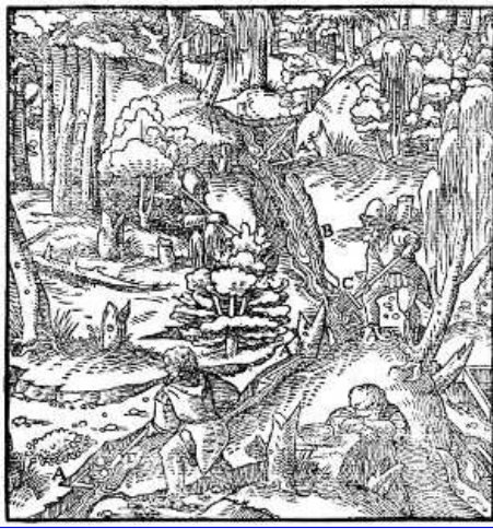
A—PITS. B—TORRENT. C—SEVEN-PRONGED FORK. D—SHOVEL. [Pg 346]
