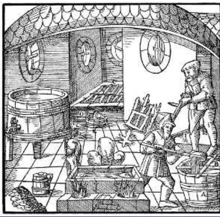
A—WOODEN TUB. B—CROSS-BARS. C—LATHS. D—SLOPING FLOOR OF THE CHAMBER. E—TUB PLACED UNDER IT. [Pg 576]
