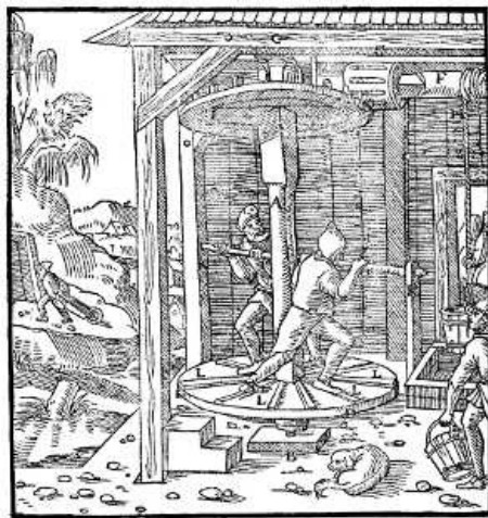
A—UPRIGHT AXLE. B—BLOCK. C—ROOF BEAM. D—WHEEL. E—TOOTHED-DRUM. F—HORIZONTAL AXLE. G—DRUM COMPOSED OF RUNDLES. H—DRAWING ROPE. I—POLE. K—UPRIGHT POSTS. L—CLEATS ON THE WHEEL. [Pg 163]
