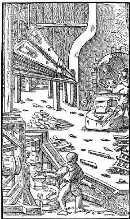
A—FORGE. B—BELLWS. C—TONGS. D—HAMMER. E—COLD STREAM. [Pg 425]
