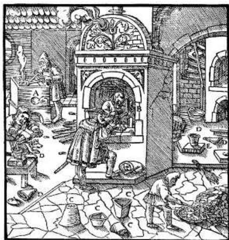
A—FURNACE IN WHICH THE AIR IS DRAWN IN THROUGH HOLES. B—GOLDSMITH'S FORGE. C—EARTHEN CRUCIBLES. D—IRON POTS. E—BLOCK. [Pg 453]
