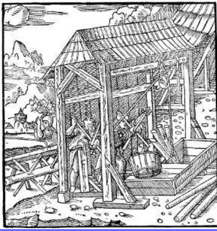
A—WINDLASS. B—STRAIGHT LEVERS. C—UPRIGHT BEAMS. D—ROPE. E—PULLEY. F—TIMBERS TO BE LOWERED. [Pg 171]
