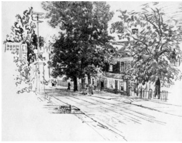
JOHNSON HOUSE, GERMANTOWN
