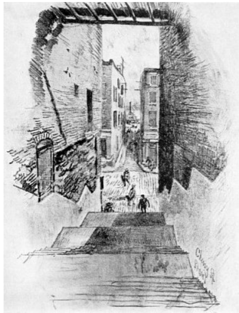
THE CHERRY STREET STAIRS NEAR THE RIVER
