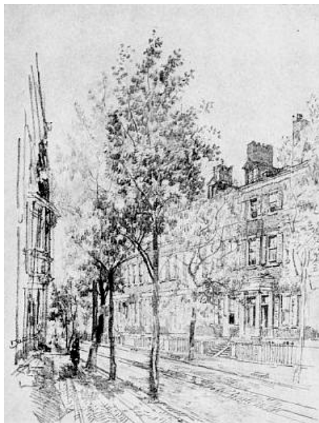
"PORTICO ROW" SPRUCE STREET
