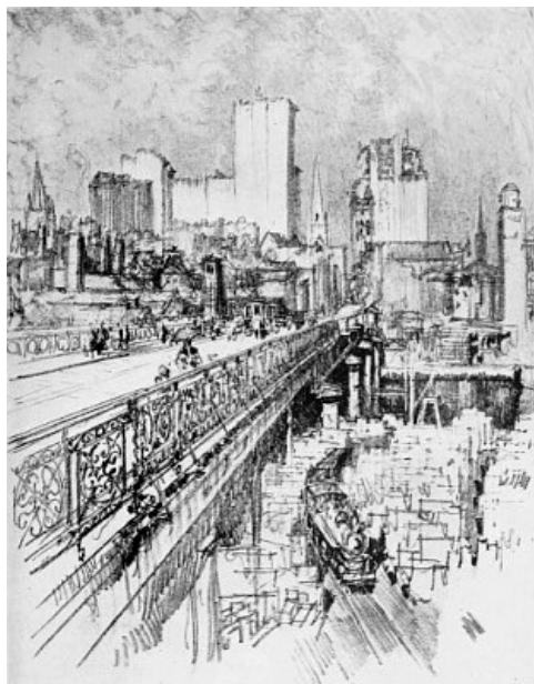
CHESTNUT STREET BRIDGE
