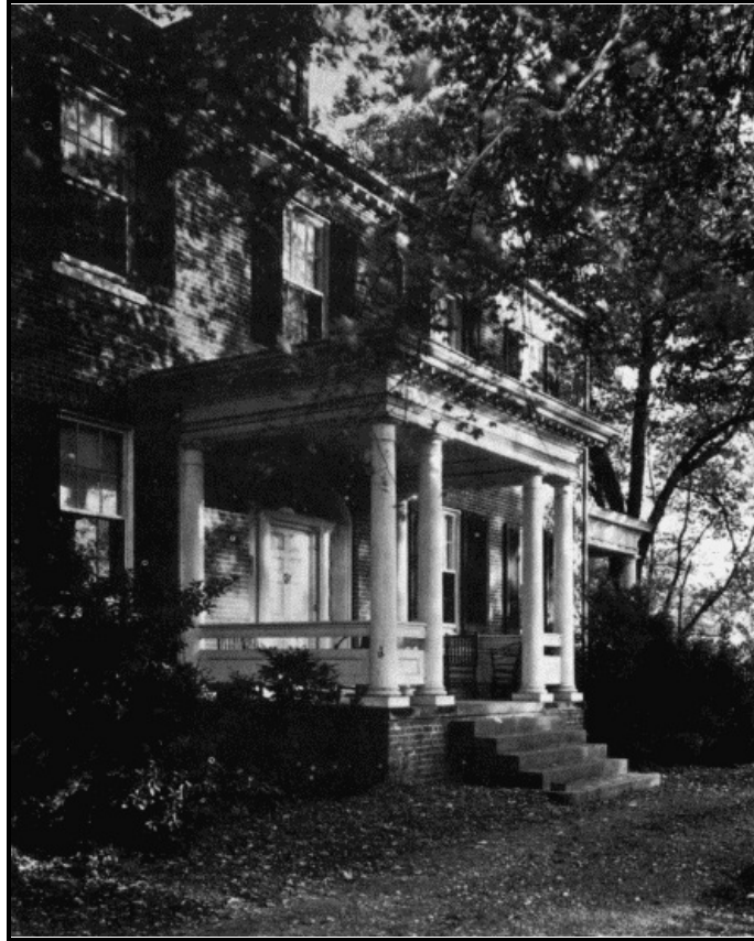
THE FRONT PORCH AT ROCKLAND, Home of the Rusts. Built in 1822 by General George Rust and still owned by his family.
