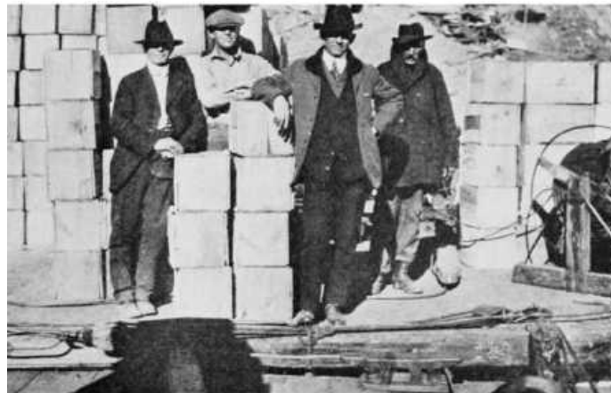
THE SUSPENSION BRIDGE AT CHELAN FALLS ( above ) OLD RIVER VETERANS ON THE LANDING AT POTARIS. (CAPT. McDERMID ON LEFT, IKE EMERSON ON RIGHT) ( below )
