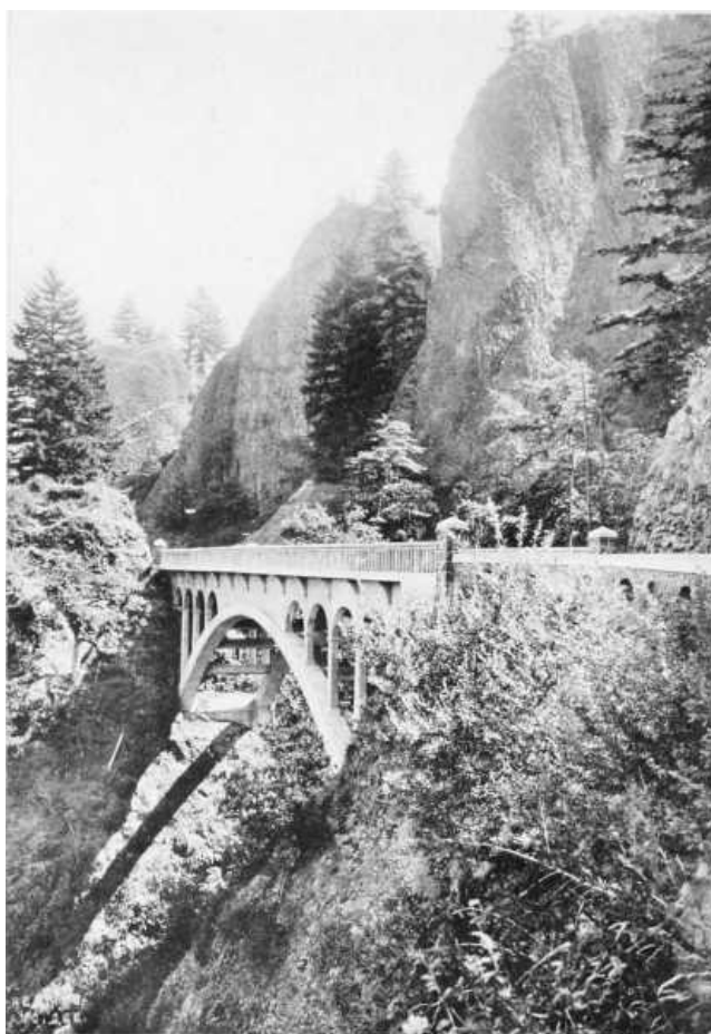
BRIDGE ON COLUMBIA HIGHWAY NEAR PORTLAND, OREGON
