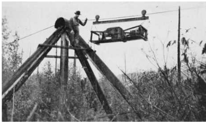
OUR WETTEST CAMP AT KINBASKET LAKE ( above ) THE OLD FERRY TOWER ABOVE CANOE RIVER ( below )
