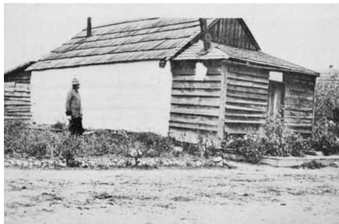
BONNINGTON FALLS OF THE KOOTENAY ( above ) PLASTERED LOG CABIN IN THE DOUKHOBOR VILLAGE ( below )
