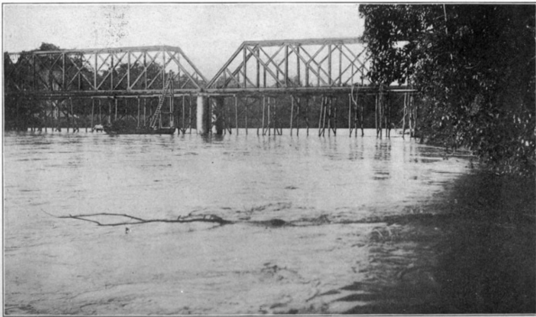
BRIDGE OVER MOTAGUA RIVER.
