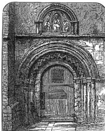
NORTH DOOR, ELSTOW CHURCH.
