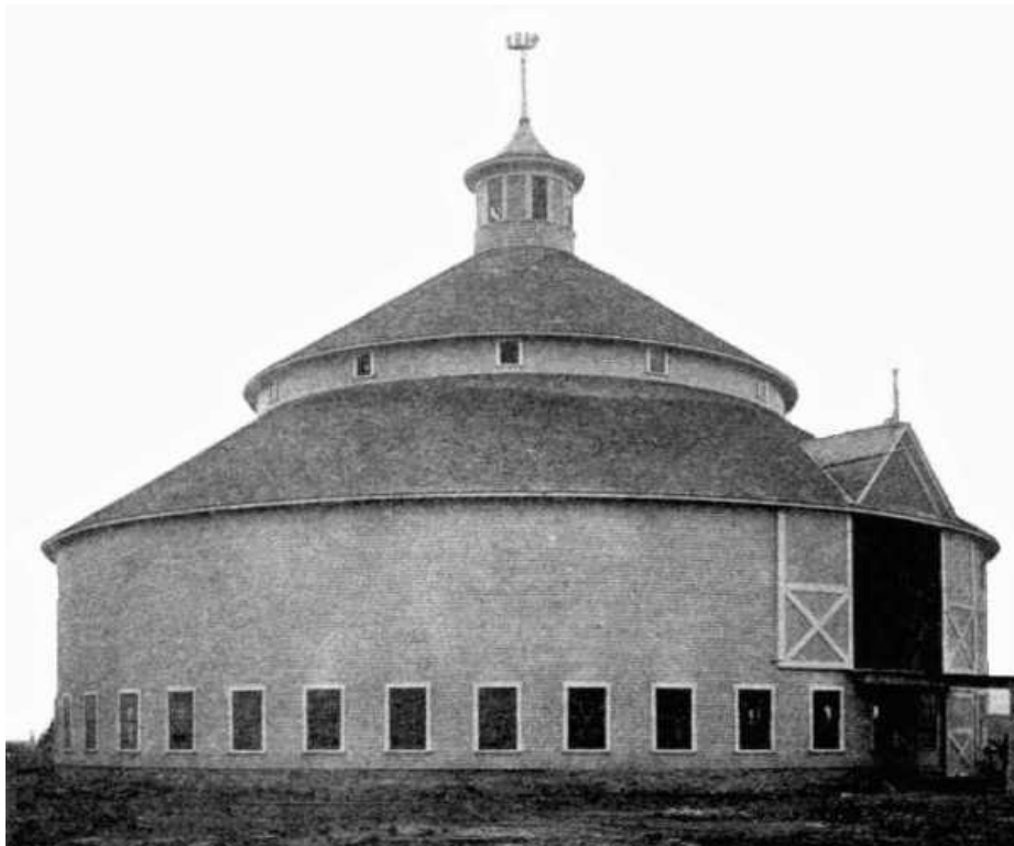
FIG. 30. BARN No. 4. 90 FEET IN DIAMETER; ONE OF THE FEW DAIRY BARN WITH SUFFICIENT LIGHT; SAME SCALE AS DRAWING ON PAGE 37 .
