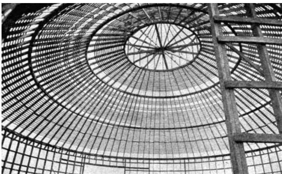
FIG. 35. VIEW OF 70-FOOT SELF-SUPPORTING ROOF ON BARN SHOWN IN FIG. 36 ; NOTE HOOPS ON STUDS IN RIGHT FOREGROUND.
