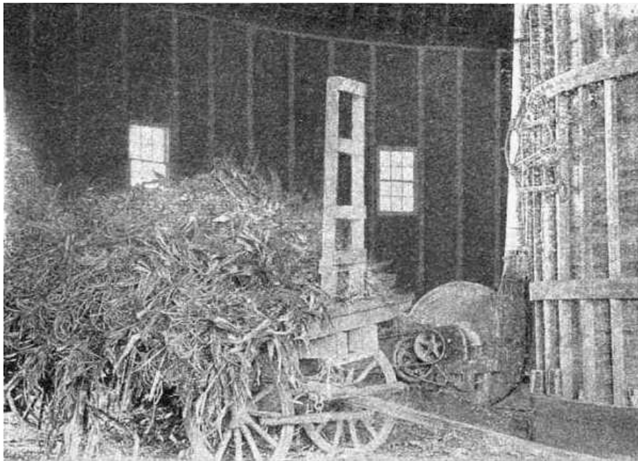
FIG. 3. INTERIOR OF BARN, SECOND FLOOR, SHOWING SILO AND LOCATION OF ENSILAGE CUTTER. (TEAM UNHITCHED TO SHOW CUTTER.)
