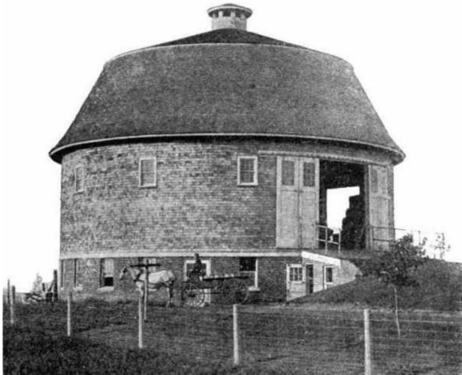
FIG. 23. NORTHEAST VIEW, SHOWING DAIRY UNDER DRIVEWAY. THE BARN IS ON THE SAME SCALE AS THE DRAWING ON PAGE 28 .
