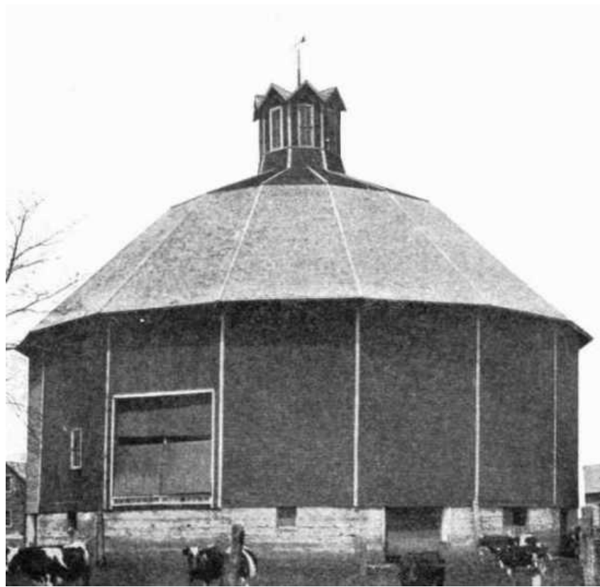
FIG. 41. BARN No. 6; 85 FEET IN DIAMETER; SAME SCALE AS DRAWING ON OPPOSITE PAGE.
