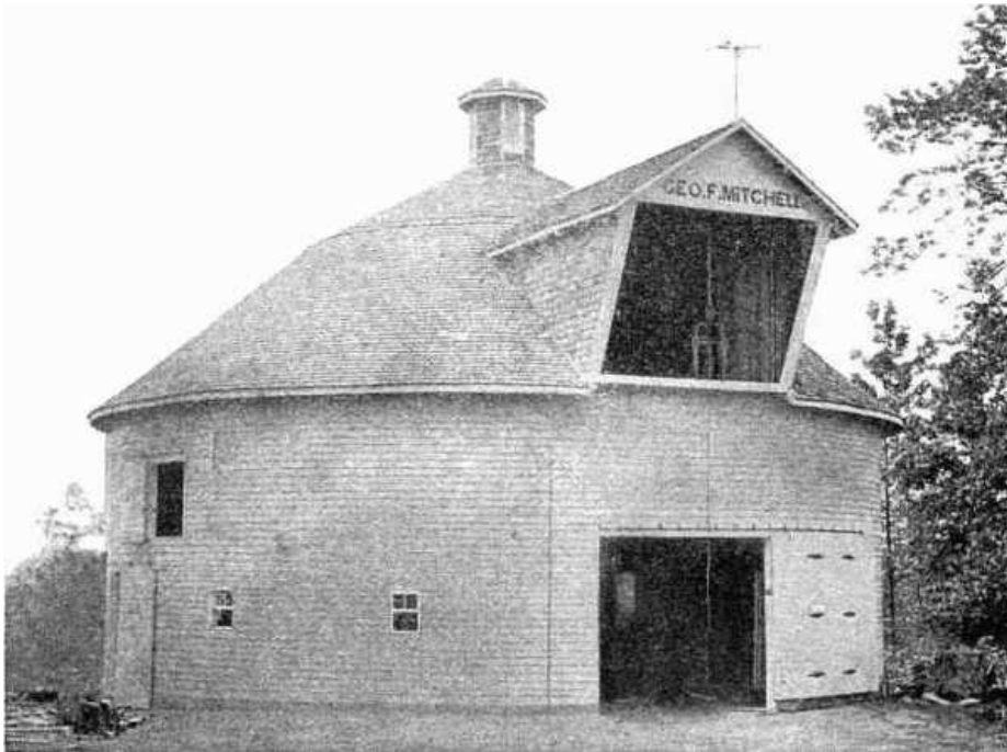
FIG. 38. BARN 48 FEET IN DIAMETER, 16-FOOT POSTS; NOTE METHOD OF TAKING HAY INTO SMALL ROUND BARN.
