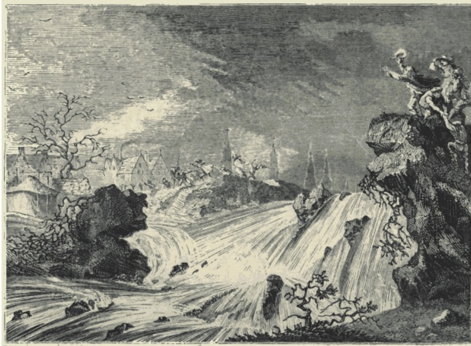
Dykes of Holland: destruction by bursting.
