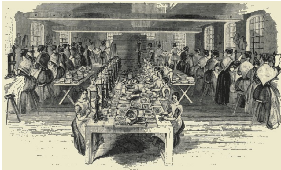
Stamping, pressing, and punching buttons.—Elliott's factory.
