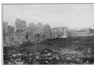
Photo: J. W. Tyrrell, October 1894. INTERIOR OF FORT PRINCE OF WALES, SHOWING WALLS OF OLD DWELLING-HOUSE
