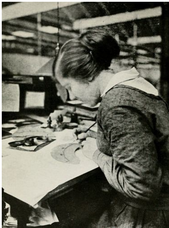
MAKING INSTRUMENT SCALES
