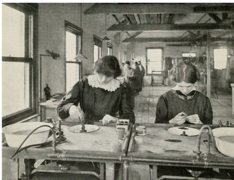
TREADLE POLISHING-MACHINES, FOR SMOOTHING LENSES
