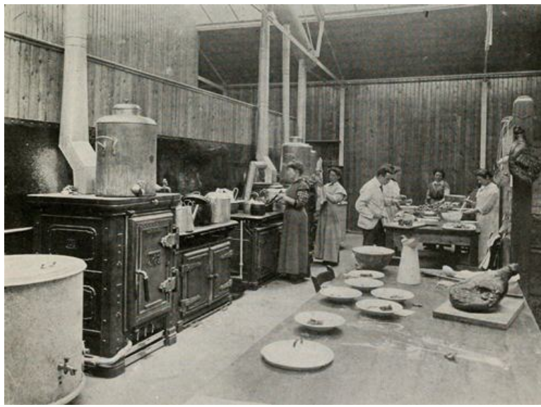
VIEW OF CANTEEN KITCHEN
