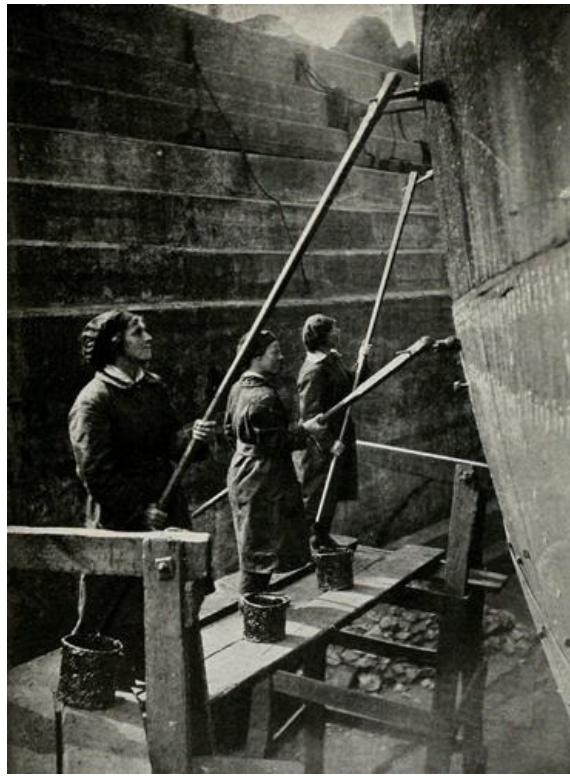
PAINTING A SHIP'S SIDE IN DRY DOCK
