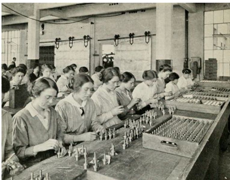
INSPECTING AND GAUGING FUSES
