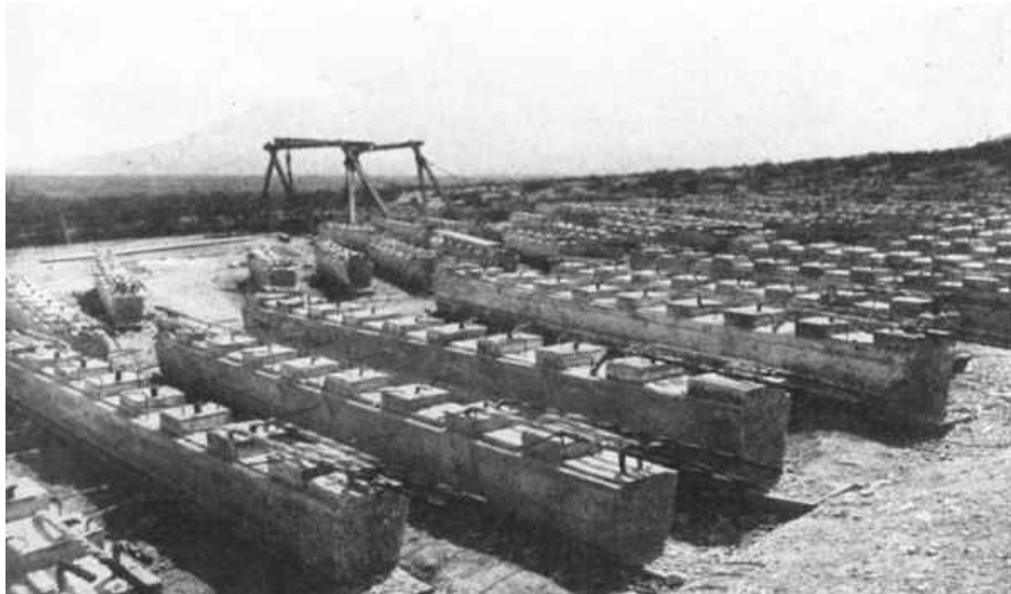
PLATE IX, FIG. 1.—VIEW OF SEPARATELY MOULDED SECONDARY BEAMS IN YARD BELOW SOUTH RESERVOIR.
