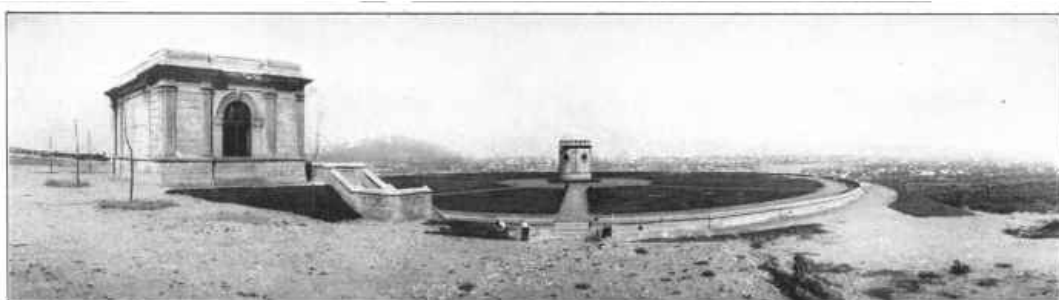
PLATE XVIII, FIG. 1.—VIEW OF SOUTH RESERVOIR, LOOKING TOWARD THE CITY.
