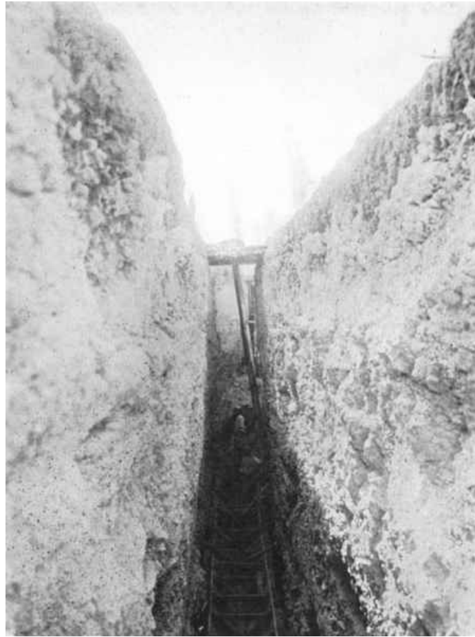
PLATE X, FIG. 2.—SETTING FORMS FOR SAN GERONIMO CULVERT.
