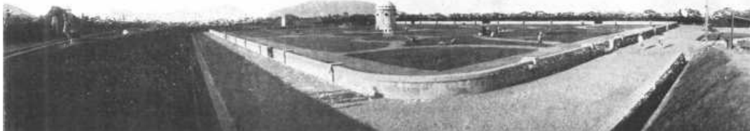
PLATE XVIII, FIG. 2.—VIEW OF ROOF OF OBISPADO RESERVOIR, LOOKING NORTH.
