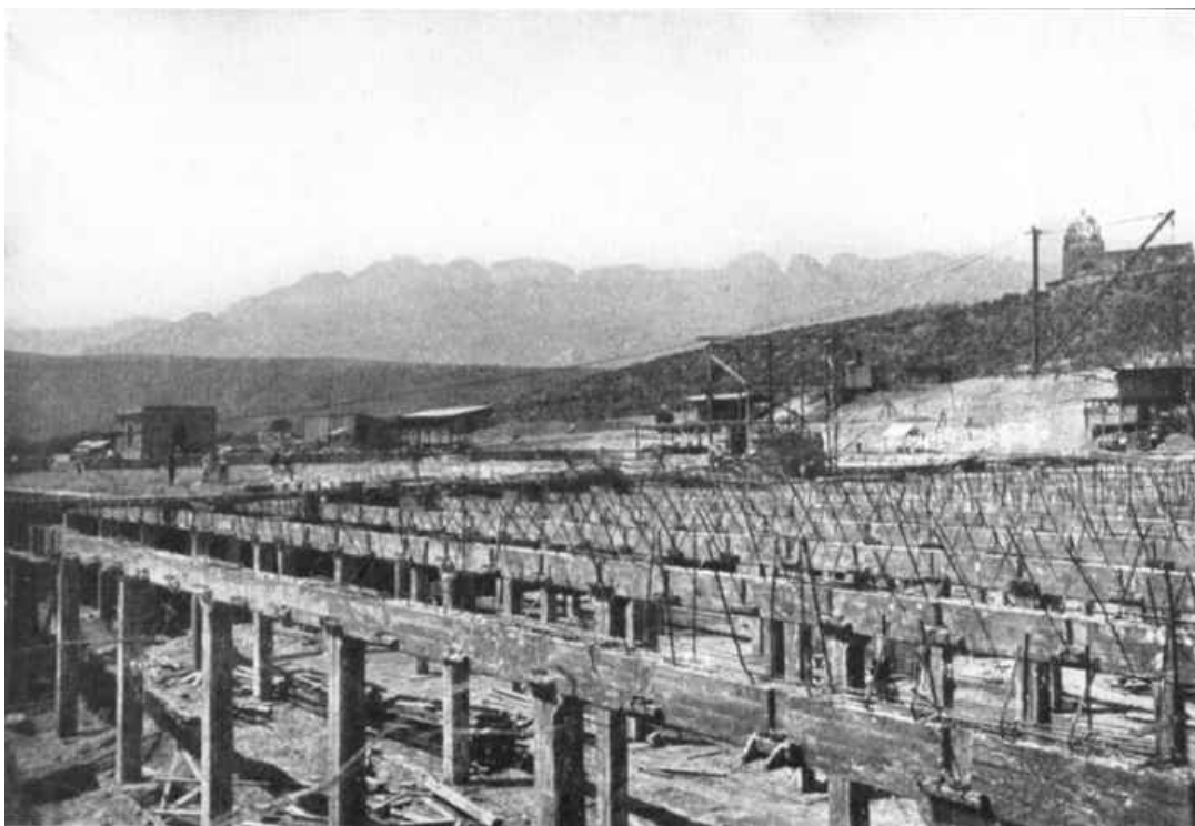
PLATE XV, FIG. 2.—PRIMARY BEAMS AND COLUMNS, OBISPADO RESERVOIR.
