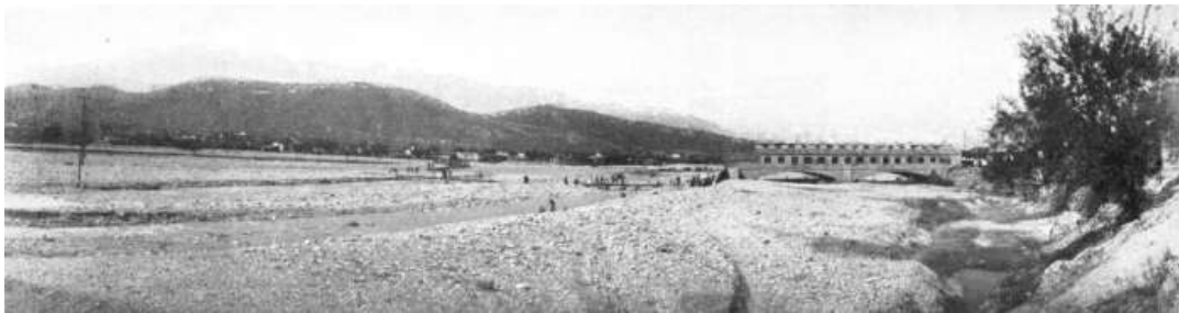
PLATE XXXII, FIG. 1.—VIEW OF SANTA CATARINA RIVER AFTER THE FLOOD.
