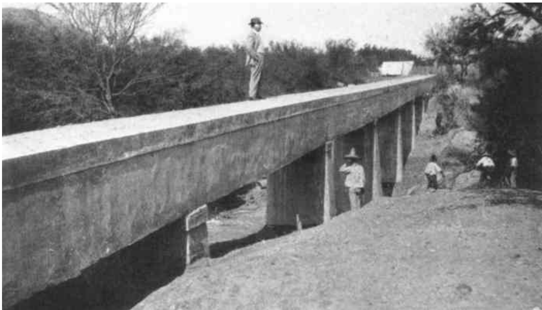
PLATE XXIII, FIG. 2.—VIEW OF ESTANCIA BRIDGE, COMPLETED.
