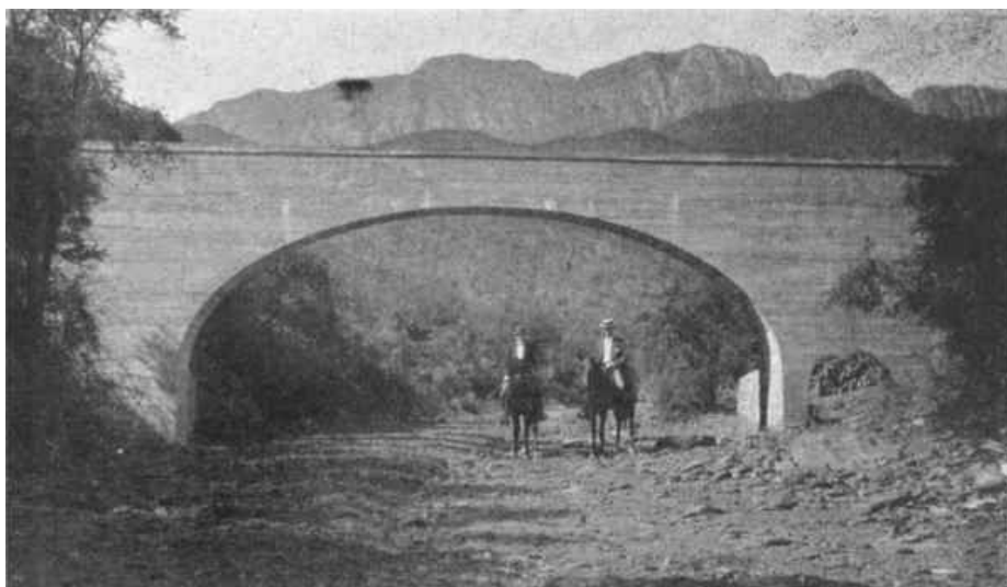
PLATE IV, FIG. 2.—ELLIPTICAL ARCH BRIDGE CARRYING ESTANZUELA AQUEDUCT.
