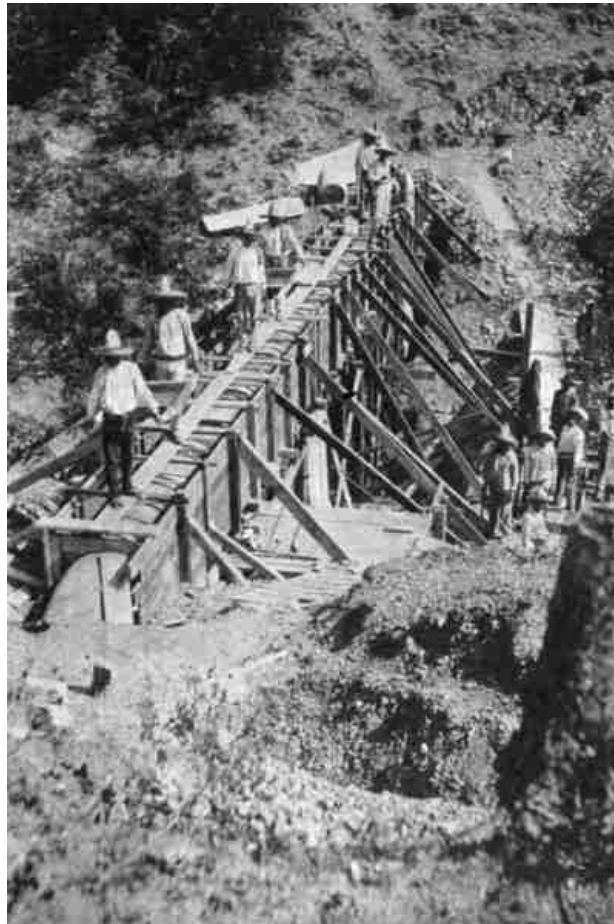
PLATE V, FIG. 2.—PLACING CONCRETE PIPES IN FORMS FOR BRIDGE CROSSING AT NORTH END OF TUNNEL, ESTANZUELA AQUEDUCT.
