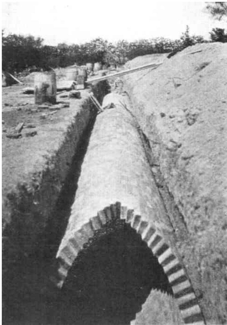
PLATE XXI, FIG. 1.—VIEW OF ARCH, OUTFALL SEWER.
