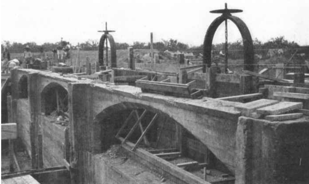
PLATE XXVII, FIG. 2.—INLET WEIRS TO LIQUEFYING TANKS, DURING CONSTRUCTION.
