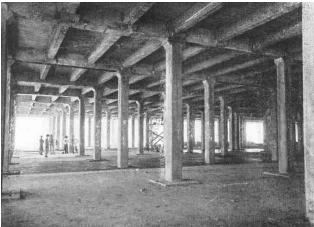
PLATE XVI, FIG. 1.—PREPARING FLOOR FOR CONCRETING, OBISPADO RESERVOIR.
