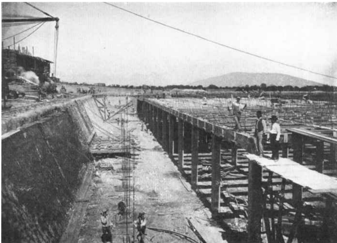
PLATE XV, FIG. 1.—CONSTRUCTION OF WEST SIDE-WALL OF OBISPADO RESERVOIR.
