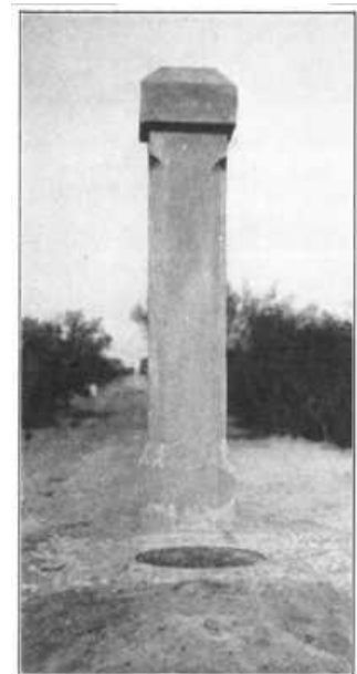
PLATE XXI, FIG. 2.— VENTILATING COLUMN AND MANHOLE, OUTFALL SEWER.
