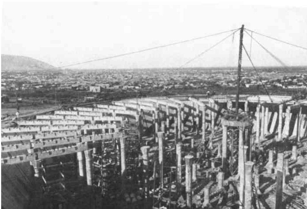
PLATE VIII, FIG. 2.—VIEW OF WESTERN HALF OF SOUTH RESERVOIR, SHOWING FINAL SETTING UP OF DERRICK ON CENTRAL COLUMNS.
