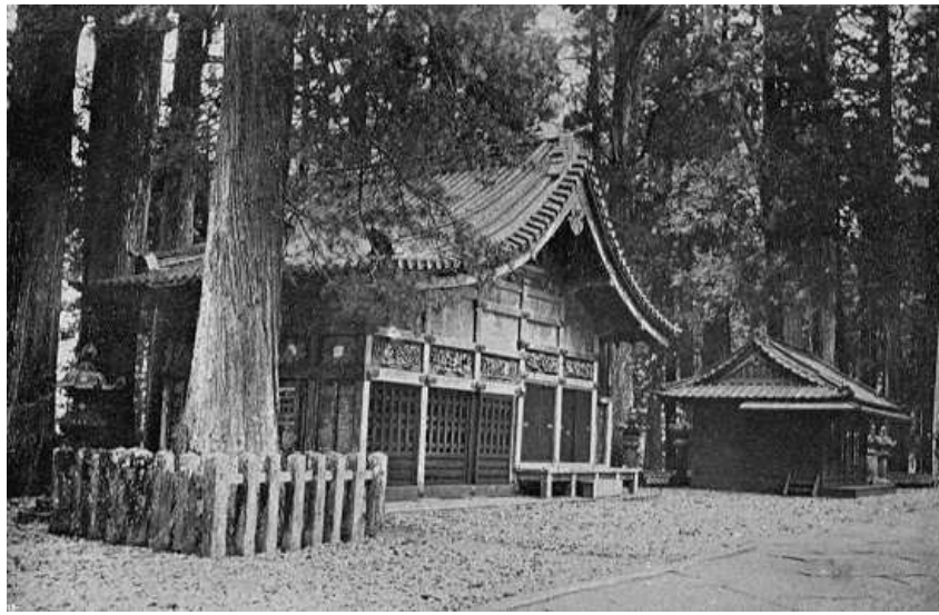
A TYPICAL NIPPON BUILDING
