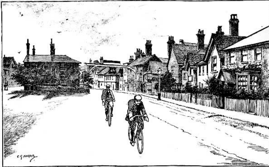
CRAWLEY: LOOKING SOUTH.
