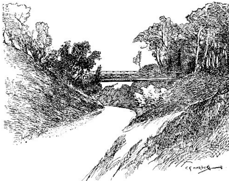
THE SUSPENSION BRIDGE, REIGATE HILL.
