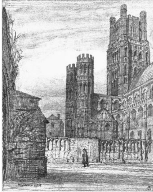
The Tower from the Cloisters.
