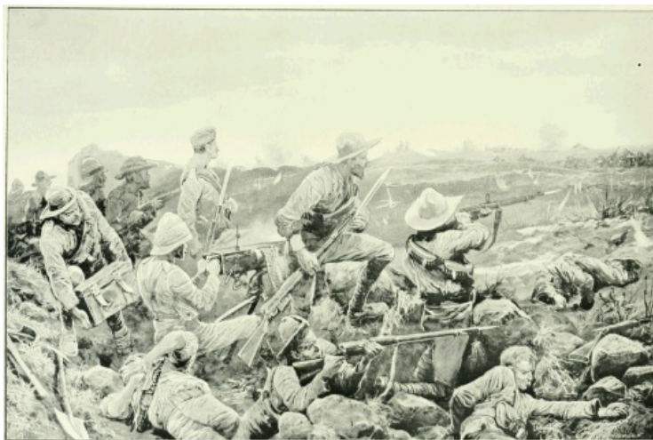
SLEEPLESS MAFEKING—HOT WORK IN THE TRENCHES.
