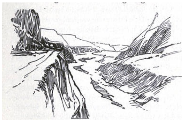
CONSTRUCTION DAYS IN CULEBRA- GAILARD CUT
