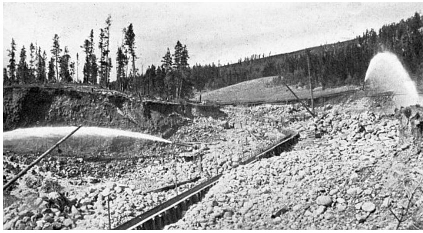
THE SNOWSTORM PLACER, FAIRPLAY, COLORADO. A TYPICAL HYDRAULIC MINE.
