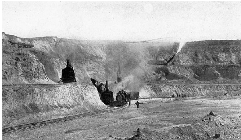
STEAM SHOVELS AND CHURN DRILLS, COPPER FLAT, ELY, NEVADA.
