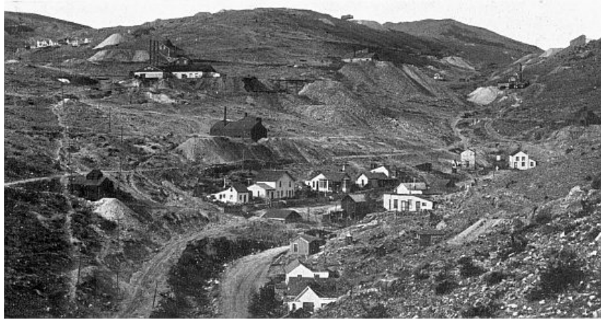
A GILPIN COUNTY, COLORADO, SCENE, SHOWING THE PRIZE, GUNNELL, CONCRETE, GOLD COLLAR, AND EUREKA MINES.
