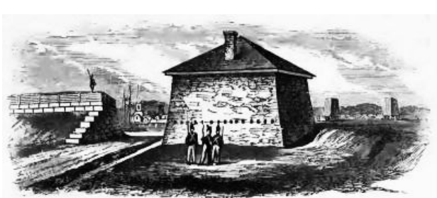
OLD BLOCK HOUSE, FORT TRUMBULL.
