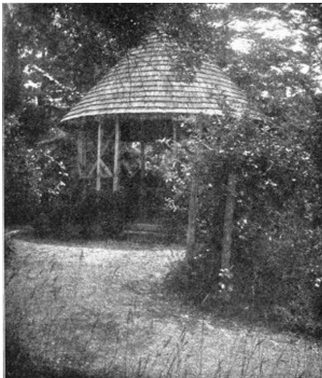
Summer-house at Ravensworth.
