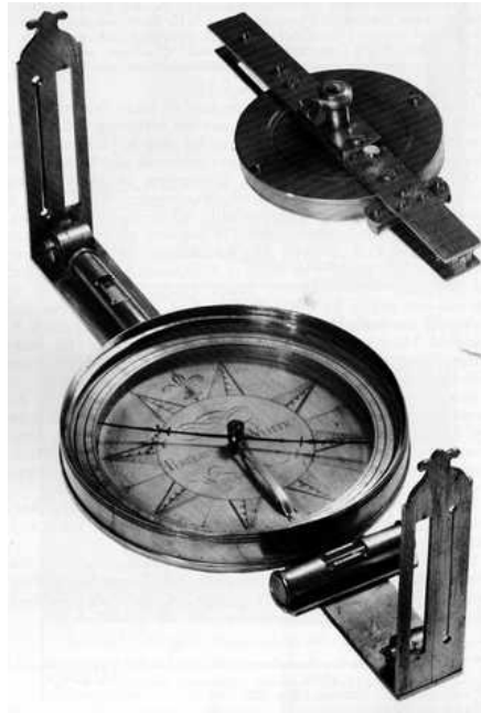
Figure 23.—Brass surveying compass made about 1790 by Peregrine White (1747-1834) of Woodstock, Connecticut. USNM 388993.
