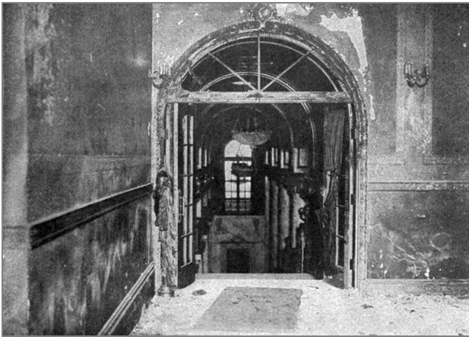
MAIN EXIT FROM FIRST BALCONY, WHERE OCCURRED THE GREATEST LOSS OF LIFE.
