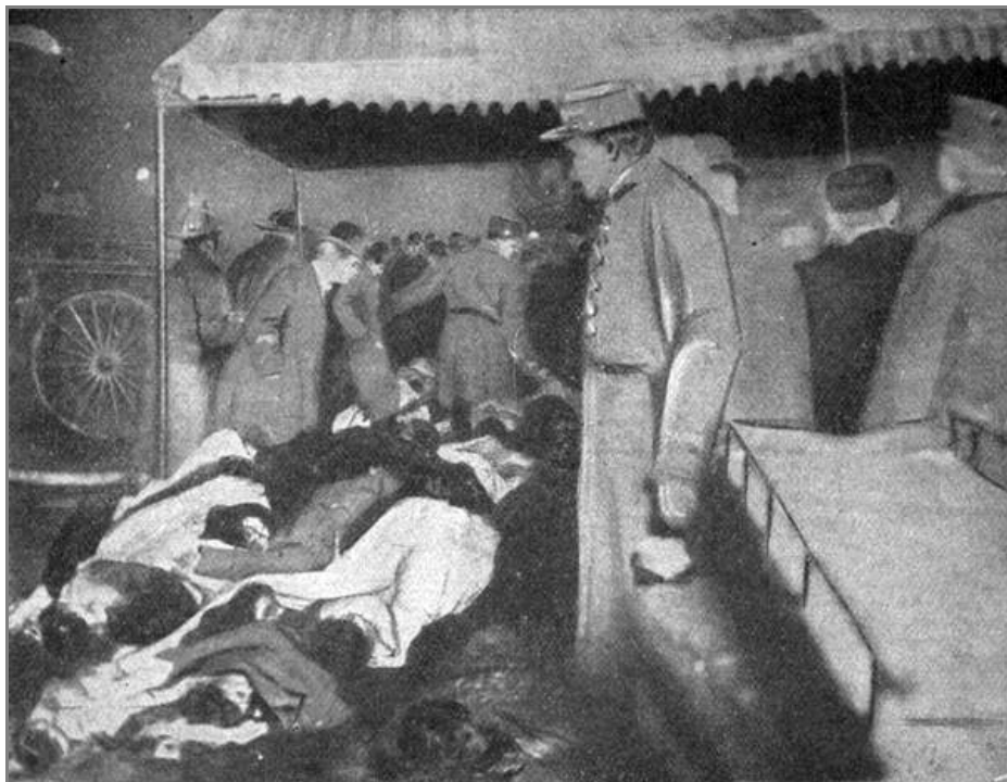
FRONT OF THEATER, PILING DEAD IN THE STREET.
