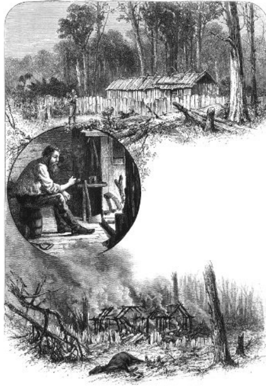
BEFORE AND AFTER THE FIRE.
