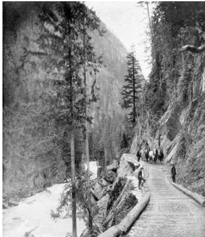
Fish River Road, in Upper Columbia Region, B. C. Photo. by Trueman, Victoria.
